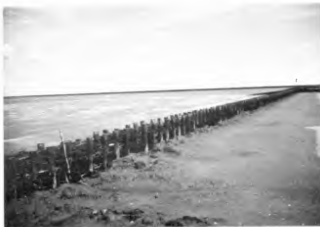
Fig. 10. Main dam with brushwood groyne (early stage).
